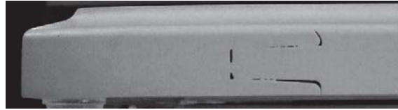
Above: Photo of joint separation at door edge
